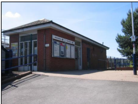
Former ticket office adjacent to platform 1 (closed October 2010)
